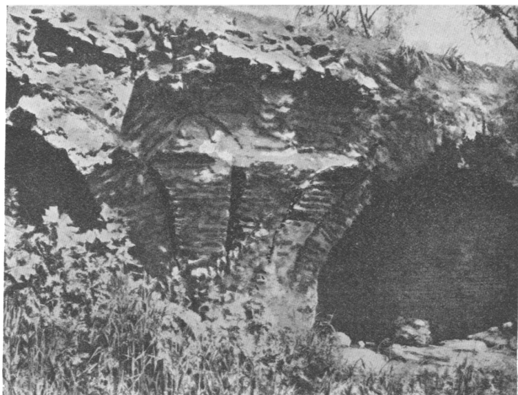
FIG. 1.—THE SPRINGING OF THE VAULTS IN ONE OF THE CENTRE COMPARTMENTS OF THE STOA.
