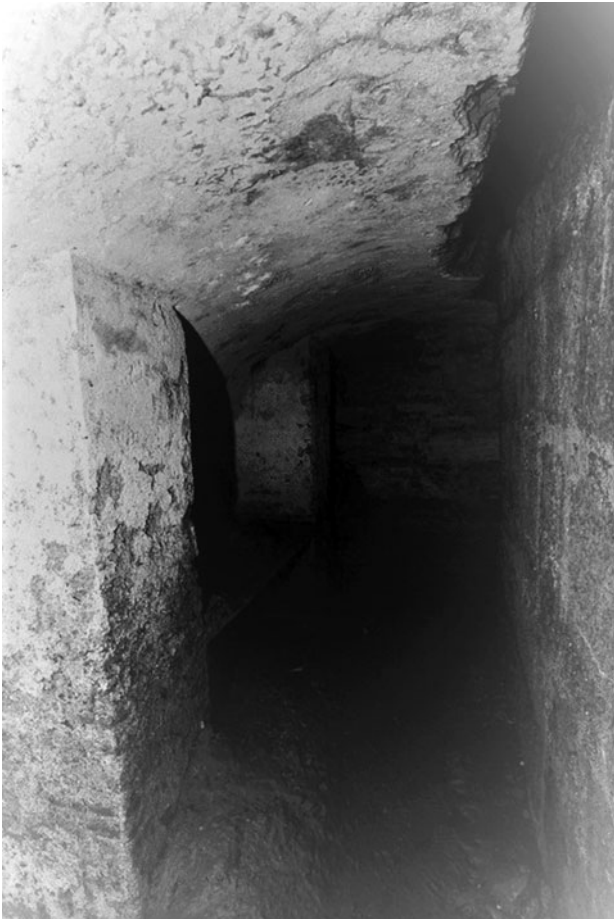
Fig. 12. The greenstone pier of the crypt breaking the north wall of the northern chamber (© Ç. Özkan Aygün).
