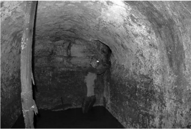
Fig. 10. Central corridor of the crypt: the masonry of the wall made of white marble blocks and, upper right, the mouth of the northwest conduit (© Ç. Özkan Aygün).
