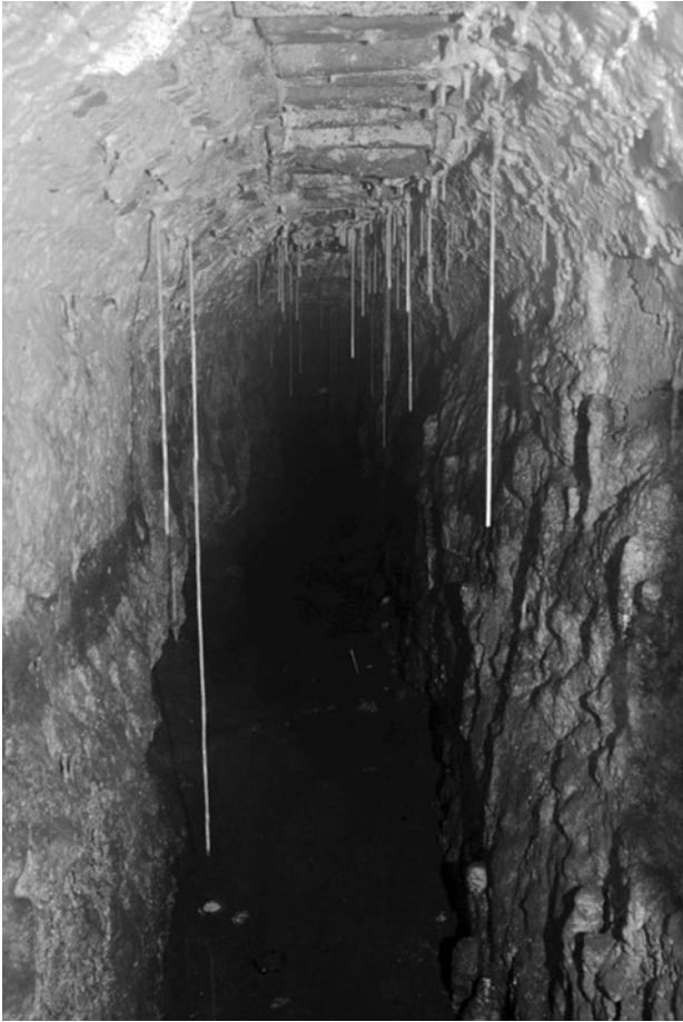
Fig. 17. Calthemites on the vault of the crypt's northwest conduit, heading west (© Ç. Özkan Aygün).
