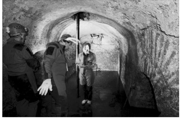
Fig. 9. Crypt. Right: double brick arches (© Ç. Özkan Aygün).
