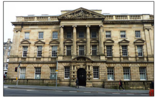
Midlothian County Buildings, King George IV Bridge, Edinburgh, Geological Survey housed here 1879-1906 (K.J. Edwards)
