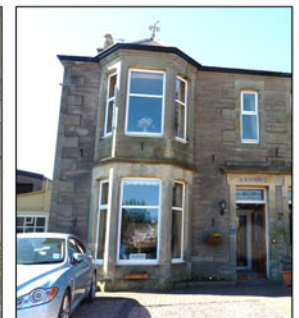
5 Pitcullen Crescent, Perth 1886-90 (K.J. Edwards)
