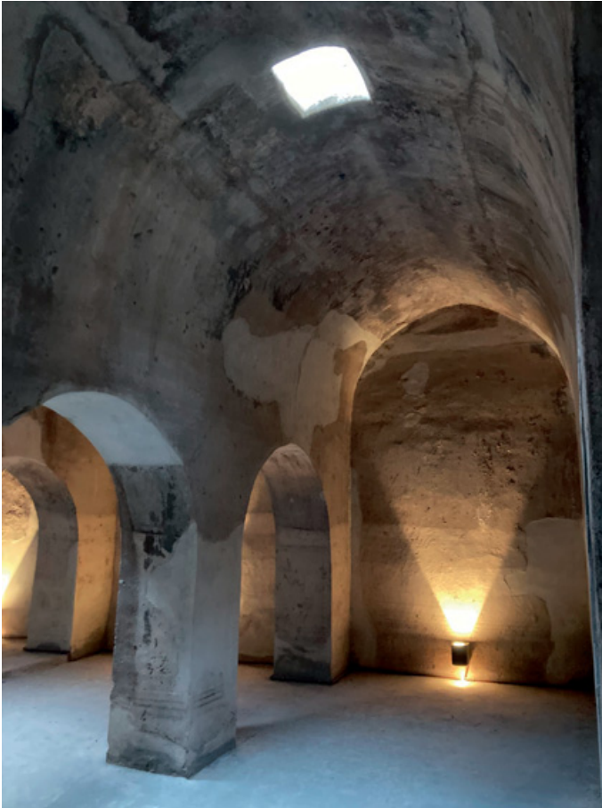
Figure 12 Barrel-vaulted interior of the Aljibe del Rey, Granada. Skylights allowed rainwater to enter the cistern during the rainy season (photo: D.F. Ruggles)
