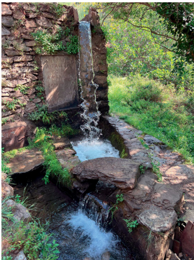
Figure 33 In the Alpujarra, as the surface canal rushing down from the mountain drops in level, a regulating basin slows its speed (photo: H. Varden)
