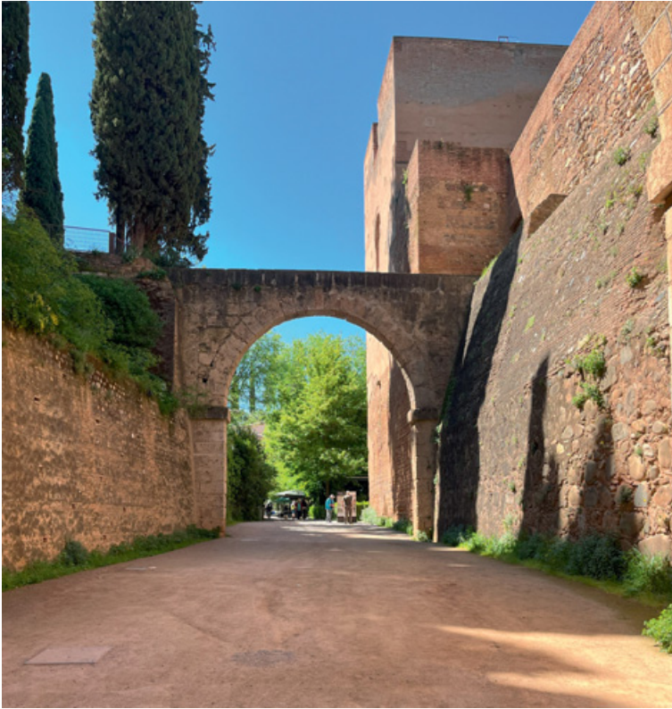
Figure 34 A one-arched aqueduct carried the canal that passes over the ravine separating the Generalife (on the left) from the Alhambra (on the right) (photo: D.F. Ruggles)
