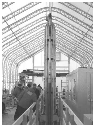
Fig. 8. Drill tower with sonde.
