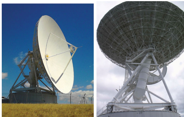
Figure 3. Photographs of the 30-m antenna after cleaning. (Images courtesy of Stuart Weston.)
