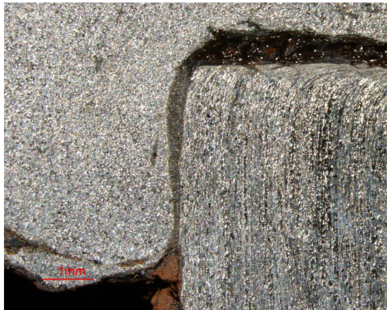
Figure. 3: Material between rivet and column.
