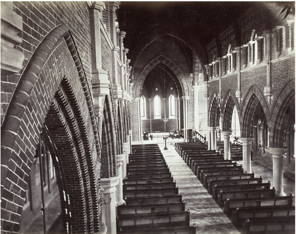
Figure 1. Interior of Holy Trinity, 1869, prior to opening, showing the quality of the bricks and bricklaying. Note: By permission of University of Bristol, Historical Photographs of China, Fr 01 -128, c2018.
