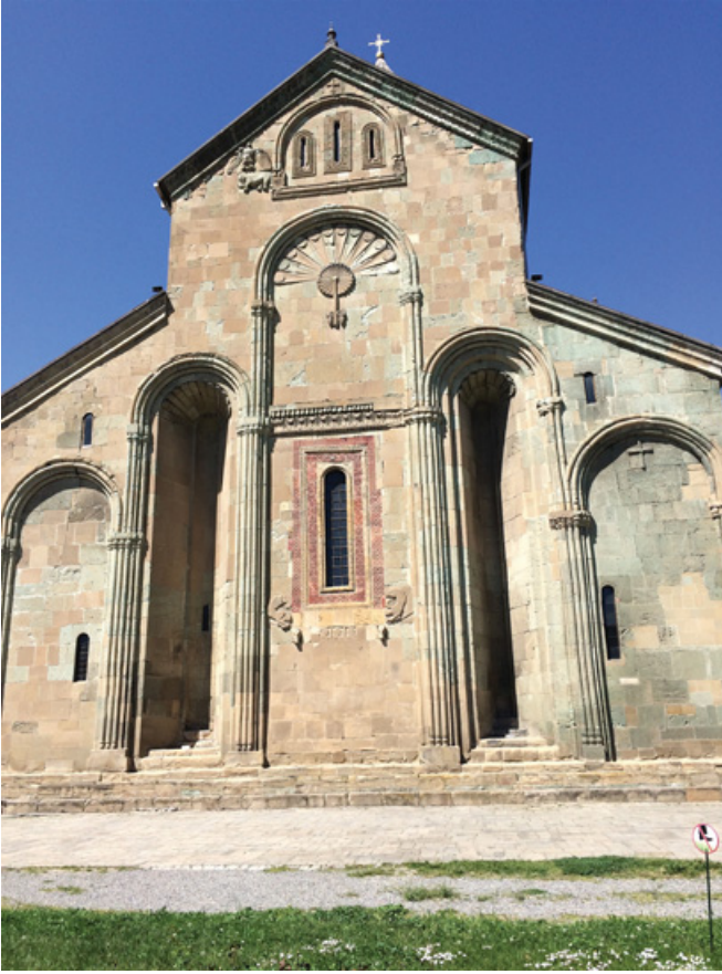
1.15. East façade, Svetitskhoveli Cathedral, Mtskheta, Georgia, eleventh century. Photograph and Copyright: Derek Krueger.
