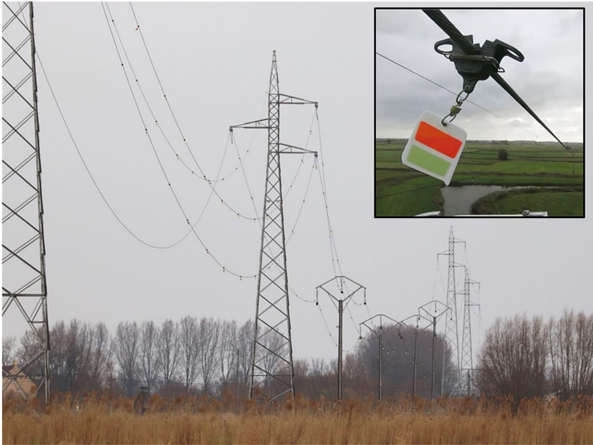
Figure 2. The study area included two pylon configurations. A taller configuration with a shield wire supported five spans at the south end, and a shorter configuration without a shield wire supported five spans at the north end. (Photo credit: James F. Dwyer.)
