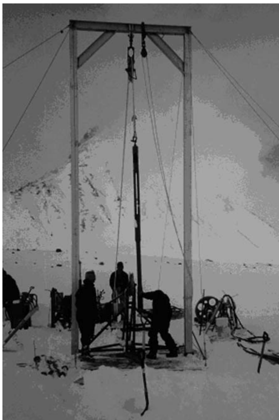
Fig. 1. Hammer and tower. The active part of the hammer slides along the slot. The hammer is hanging from the tower in the extended position, the position it would have at the bottom of the hole at the moment of impact when hammering up.
