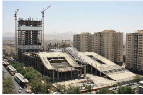
Figure 7. Unfinished Megāpārs multifunctional shopping center. Photograph: Internet. https://es.pinterest.com/pin/403846291565693866/ .
