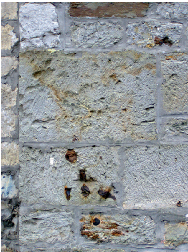
Fig. 3. St Medardus church at Vreeren, showing large chiselled blocks of 'Elst tauw' containing dark flint nodules, displaying rusty brown weathering colour due to alteration of pyrite which is mostly concentrated in the flint nodules.
