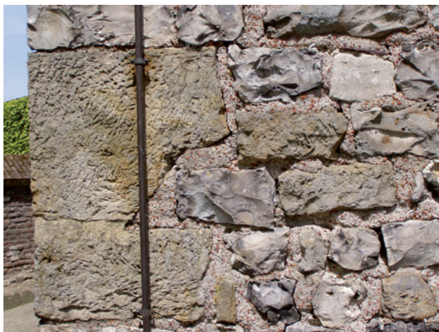
Fig. 2. St Servatius church at Sluizen, showing large chiselled blocks of 'Elst tauw', adjacent to normal-sized flint blocks.
