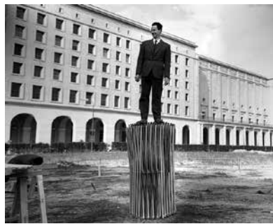
1 Emilio Pérez Piñero standing on top of one of the 'bundles', which, retracted would for easy transportation, would cover a large surface area.
