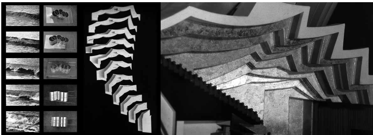
8 The acoustic ceilings for the Opera House, which were destined never to be built, were inspired by rolling waves. Recent computer modelling in Australia suggests that they would have been close to perfect acoustically
