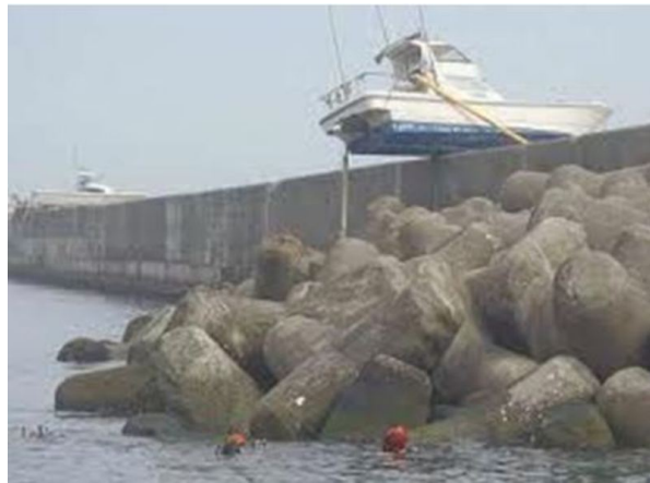
In Tohoku, seawalls and tetrapods were overwhelmed
